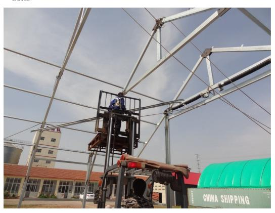
Fix D2 by No.D34, D30, D32. Fix No.D1 3" side track & vertical track to upright. Connect No.D2 and No.D1 by No.D33
