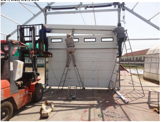
Now the installation for overhead door is completed.
